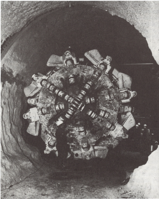
FIG. 2--View of 4.5 metre diameter 'Robbins' boring machine.
